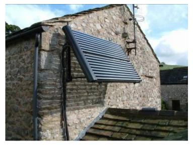
Figure 5.2 - Evacuated Tube Collectors - West Barn, Malham
