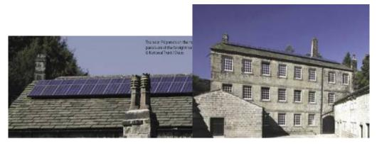
Figure 6.1 – Close up and ground level photo of PV Array on Gibson Mill, Grade II listed building
