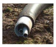
system, which is a well-insulated pipe running from the boiler accumulator tank across the site (see above right), with connections for each residence. It is possible to monitor each residences heating demand from the system by means of a heat meter, which can be used to bill each householder on the proportion of heat they use.
