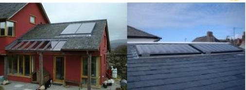
Figure 5.1 - 4m<sup>2</sup> Roof Integrated Filsol Flat Plate Collector
