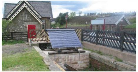
Figure 5.3 – Freestanding SHW array Dent Station, Settle - Carlisle Railway Conservation Area
