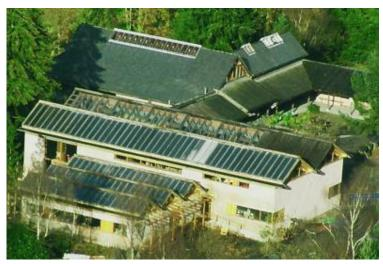
Figure 5.4 – 112m<sup>2</sup> drainback solar thermal system on Ateic building at CAT
