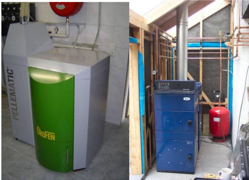
Figure 5.8 – Okofen and Baxi pellet boiler systems, as installed
