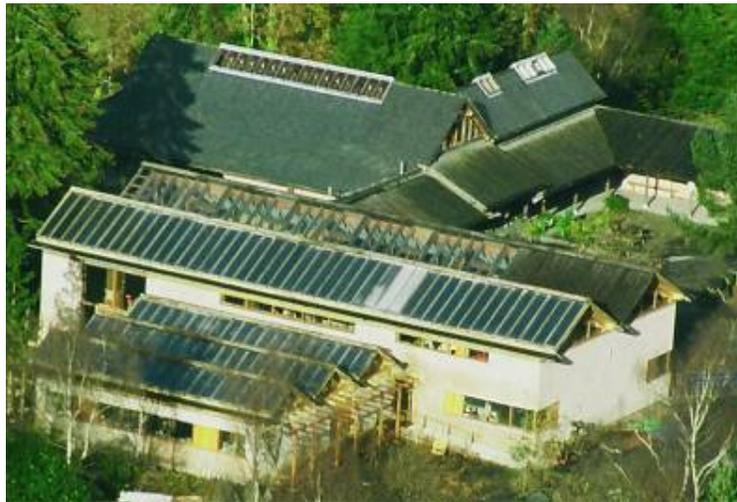
Figure 5.4 – 112m<sup>2</sup> drainback solar thermal system on Ateic building at CAT
