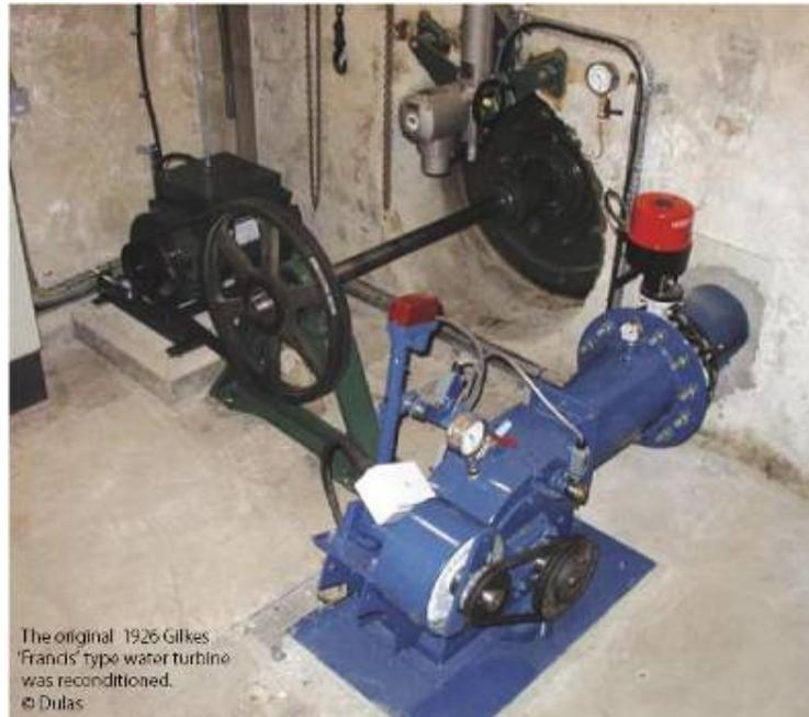
Figure 6.8 – 9kW Francis turbine at Gibson Mill – low head site
