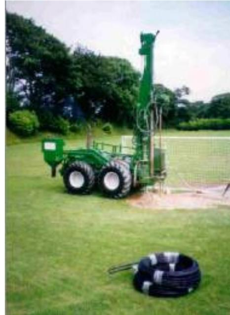
Figure 5.5 – Slinkys and boreholes for GSHP heat exchanger loops
