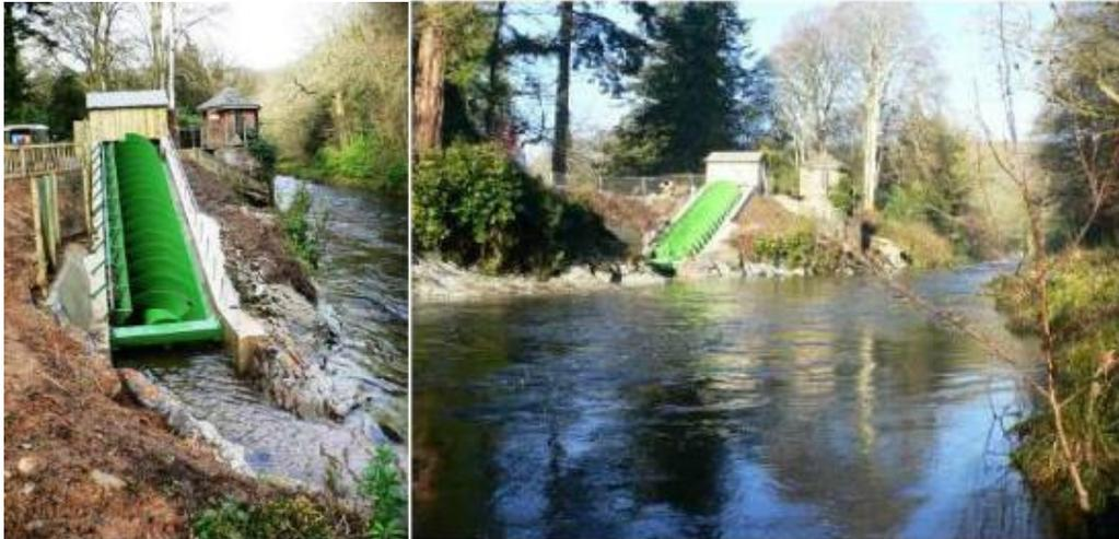
Figure 6.9 – Archimedes screw hydro turbine on the River Dart
