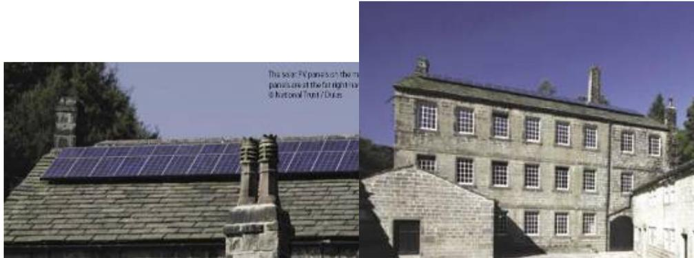
Figure 6.1 – Close up and ground level photo of PV Array on Gibson Mill, Grade II listed building
